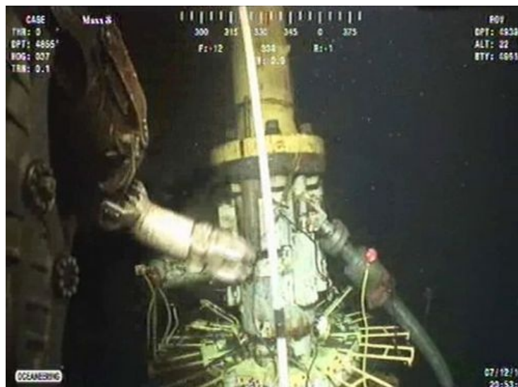
An ROV placing a cap on a wellhead.
