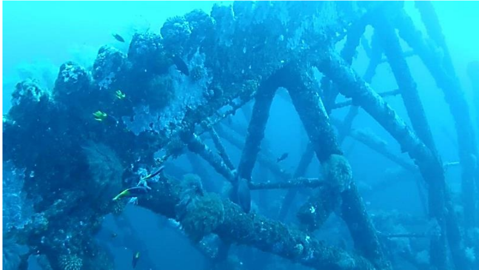
An artificial reef created from an obsolete oil and gas platform in the Gulf of Mexico.
