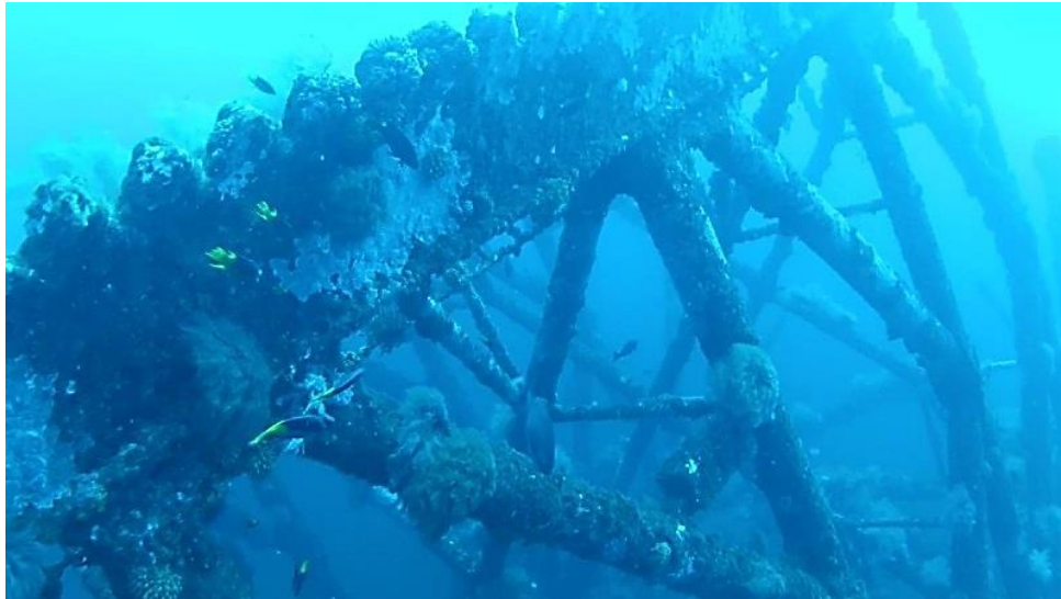
An artificial reef created from an obsolete oil and gas platform in the Gulf of Mexico. Photo credit: State of Louisiana, Department of Wildlife and Fisheries, Artificial Reef Program.
