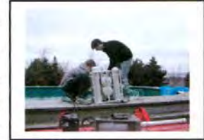
Fig. 5-1: Checking for leaks.
