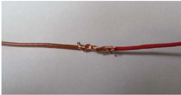
Photo #1: Two wires stripped and twisted together
